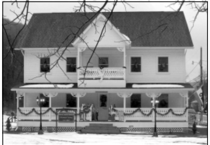
Restored Edward O. Austin's home - museum and the home of the Historical Society
